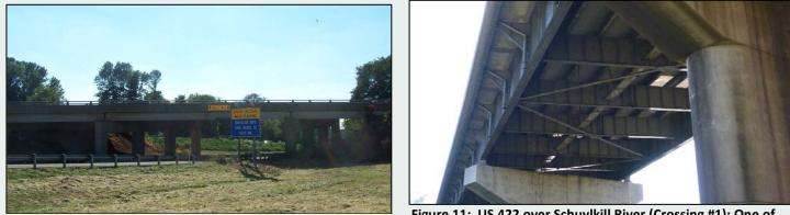
Figure 10: Perkiomen Avenue over US 422 Westbound; Functionally Obsolete Due to Substandard Clearances
