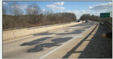
Figure 9: US 422 over Brentwood Drive; Structurally Deficient due to Deck Condition
