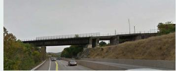
Figure 16: Two-Track, Dual Girder Railroad Crossing 2
