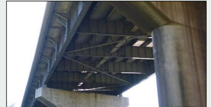
**Figure 11: US 422 over Schuylkill River (Crossing #1); One of Five Non-Redundant Fracture Critical Structural Systems**
