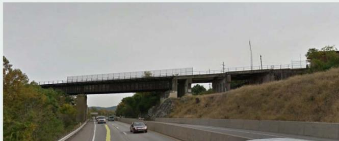
**Figure 16: Two-Track, Dual Girder Railroad Crossing 2**
