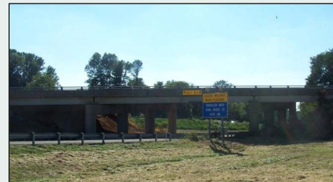
**Figure 10: Perkiomen Avenue over US 422 Westbound; Functionally Obsolete Due to Substandard Clearances**
