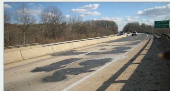
**Figure 9: US 422 over Brentwood Drive; Structurally Deficient due to Deck Condition**
