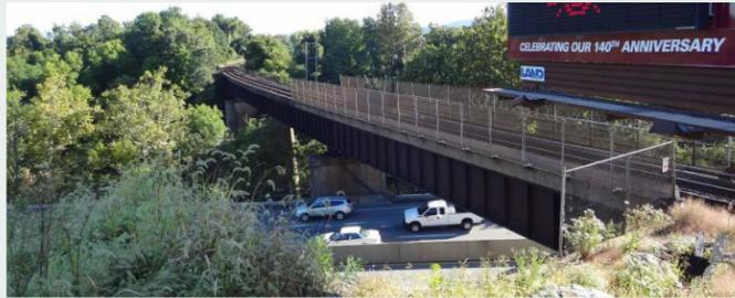
**Figure 15: Single Track Dual-Girder Railroad Crossing 1**
